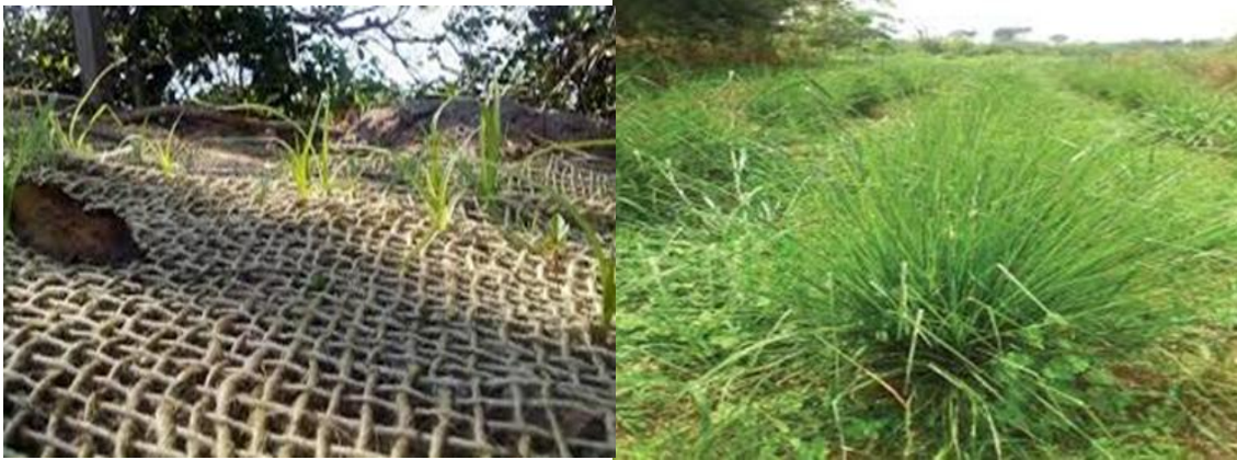
Fig. 1 Vegetative Cover with jute mat[4]
