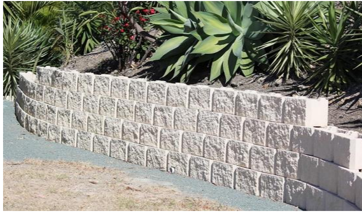
Fig. 6 Retaining Walls and Riprap
