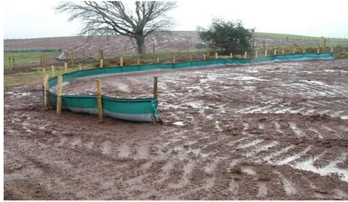
Fig. 7 Geotextile sediment fences targeted to catch sediment from cultivated land on slopes.
