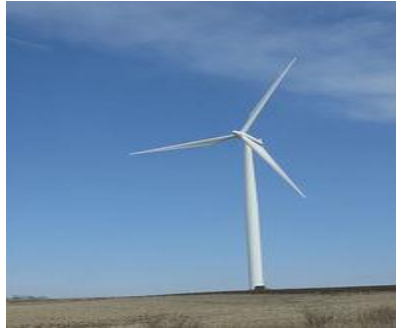
Fig. 4. A wind turbine. The Betz limit gives the maximum amount of power it can convert into motion and electricity [12].
